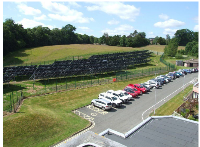
Solar PV Panels at Borders General Hospital
